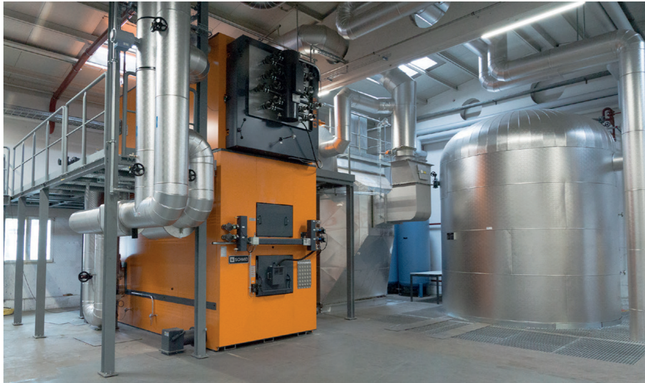
Schmid - Moving grate boiler UTSR-1600 visio
